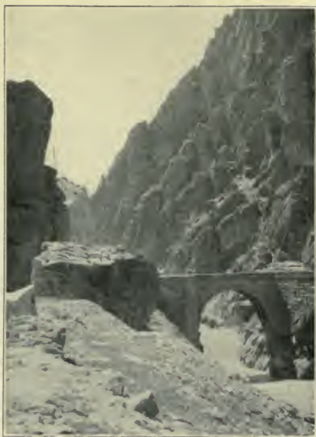
IN THE GORGE OF EL KANTARA, OLD ROMAN BRIDGE, RESTORED
