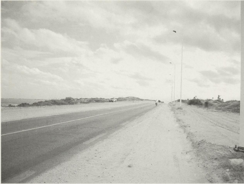
Photo 5 – The site of Ghizène in 2006, with road track cutting the settlement hill, viewed to the north-east (photo S. Ben Tahar).
