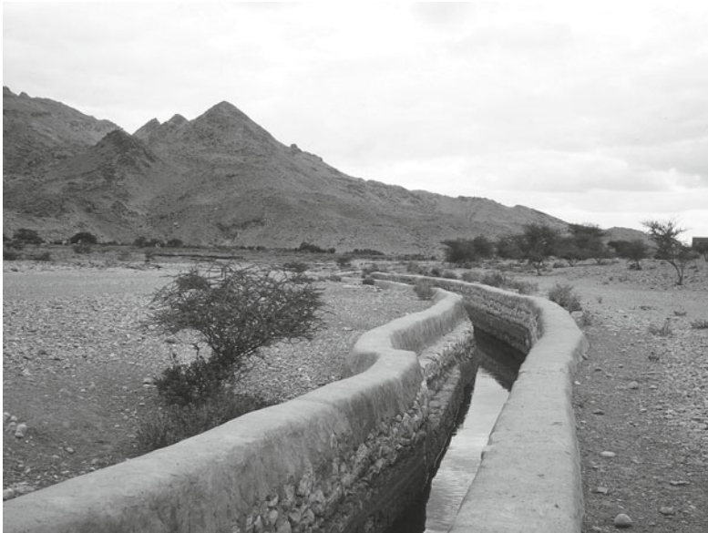
Figure 1.4 A falaj or water distribution system in the governorate of Dakhiliyah, combining human ingenuity with social organization
