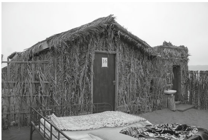
Figure 1.3 Barasti hut, constructed of native palm fronds, provides shelter from the wind and sand in the desert regions of Oman
