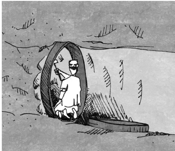
Fig. 5.10 A worker using the technique of Pish-Kaval
