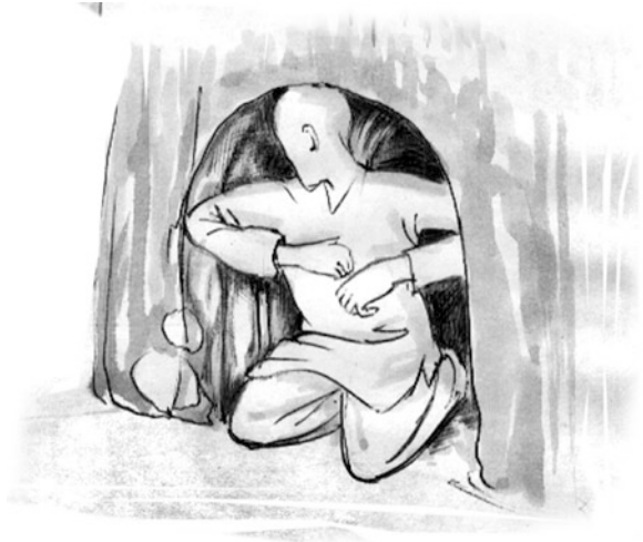
Fig. 4.11 The workers use their forearms to measure the width of tunnel
