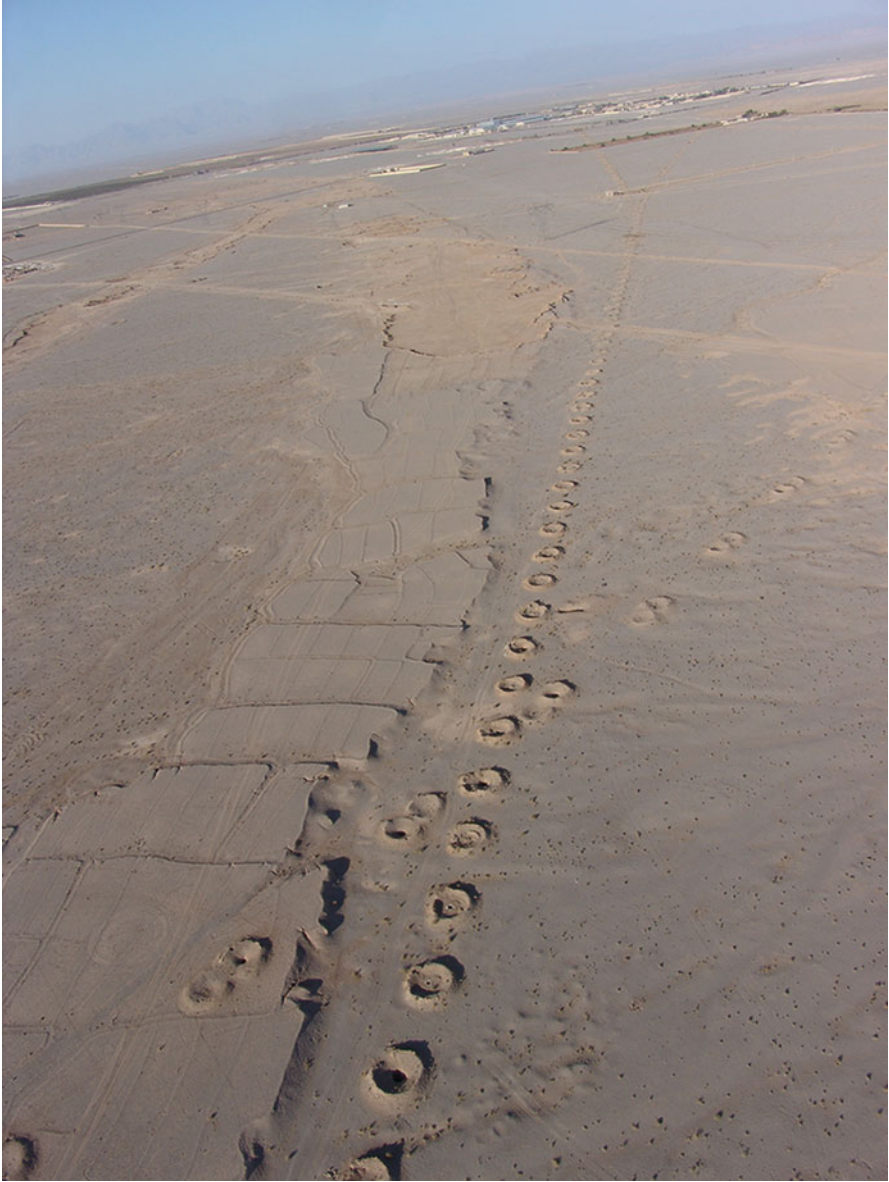
Fig. 1 Two intersecting qanats near the town of Meybod, Yazd Province, Iran (Photo by Mehdi Khebredest)
