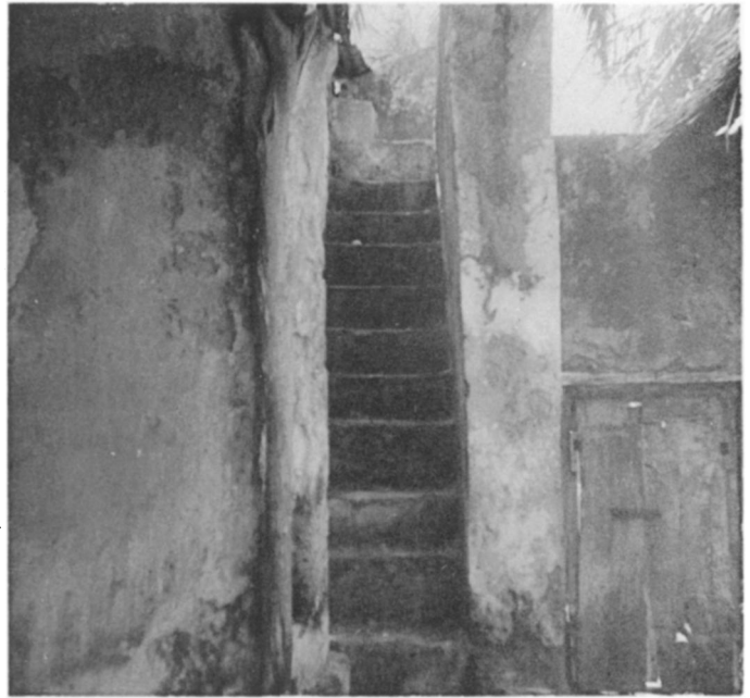
FIG. 2.—BAGAMOYO, GREAT MOSQUE, STAIRCASE MINARET.
