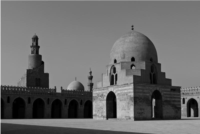
Figure 1.1 The Mosque of Ibn Tulun. (Source: Getty Images UK)
