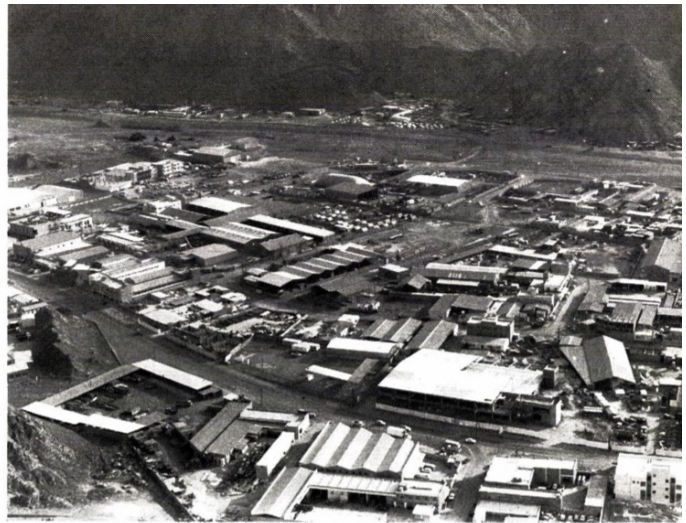
Light industries, assembly and fabrication shops, and showrooms have expanded (above) on the western edge of greater Matrah
